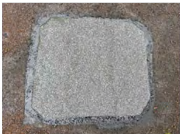
All cores sealed using a felt cap sheet
