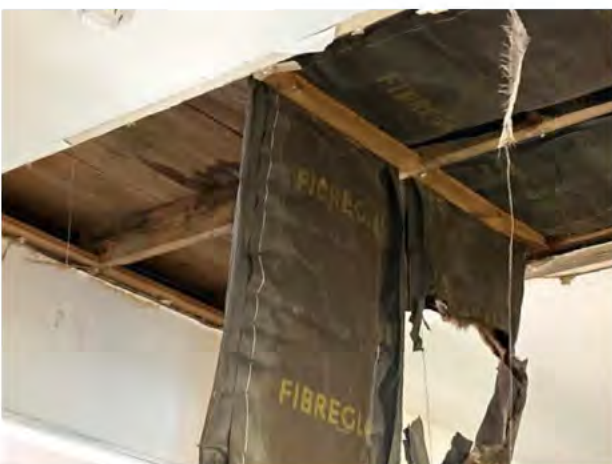
Timber T&G decking confirmed from the internal survey
