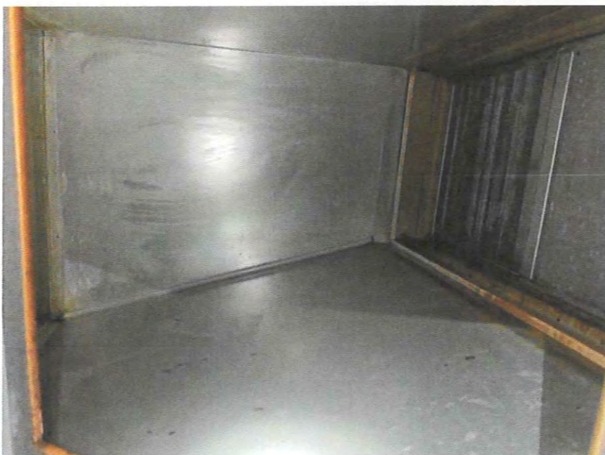
Duct upstream of fan - After Clean
