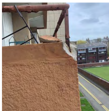
Spalling on the balcony.
