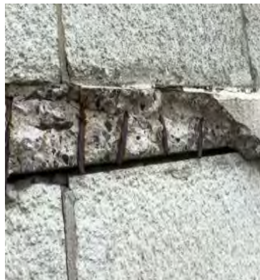
Spalling and exposed rebar on the string course
