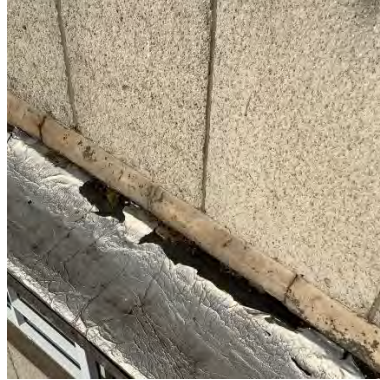
Previous flash band repairs.
