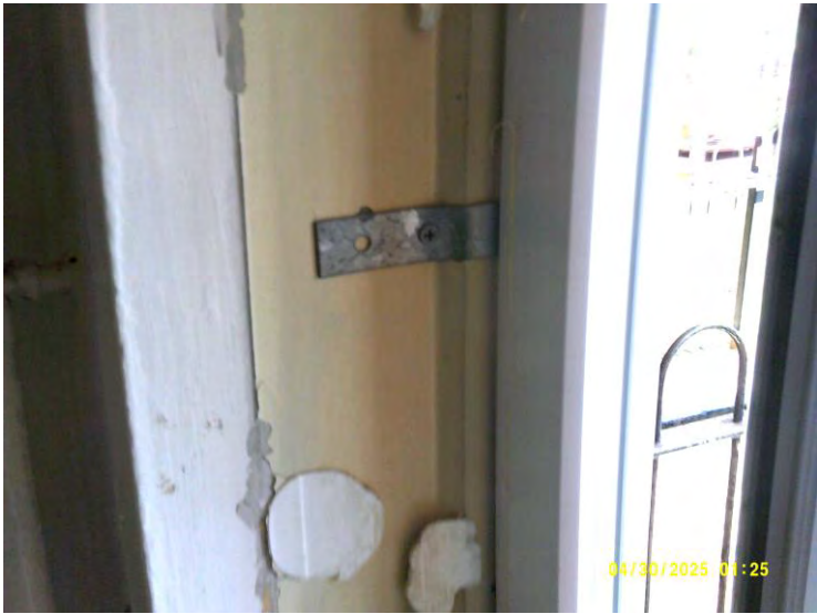
Typical Window Frame Connections
