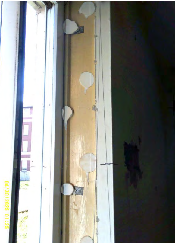
Typical Window Frame Connections
