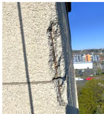
Spalling and exposed rebar on the Orlit panel
